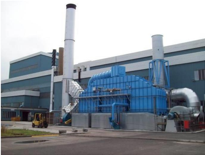
**Oxidiser** – 3 canister RTO destroys over 99.5% of the solvent, and captures the heat with enough solvent the oxidiser requires no additional gas.
